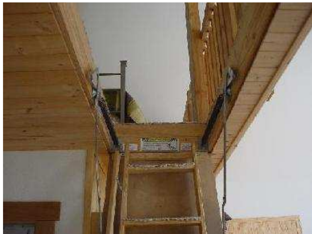
Looking up at loft access
