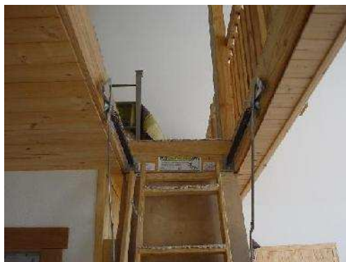
Looking up at loft access
